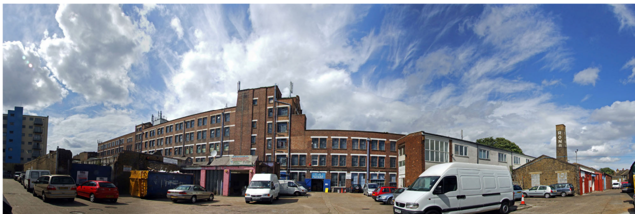
Copeland Industrial Park – huge potential for new public realm, mixed rehabilitation and new buildings
