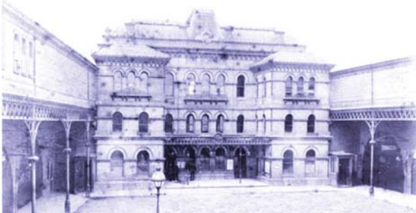
Peckham Rye station frontage in late C19th (Photo by RLSAG)
